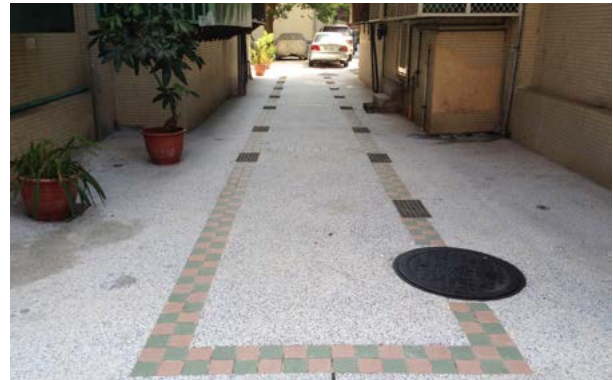
► Post-construction of user drainage equipment project for sewage.
