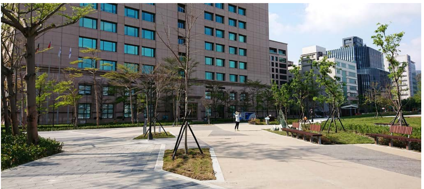
► Water-permeable sidewalk at Gangqian Park.
