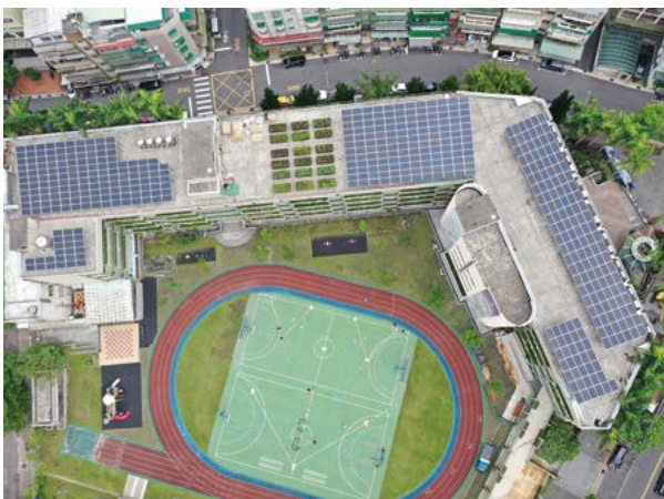
► Installation of 146.4kW at Wan Xin.
