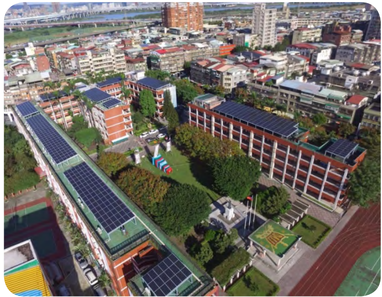
▲ Installation of solar photovoltaic system on school rooftop
