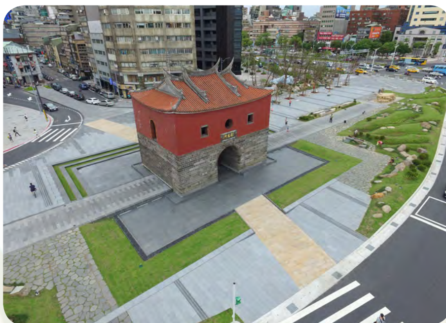
▲ Permeable pavement at the North Gate Square
