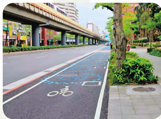
▲ Permeable pavement on bike lanes
