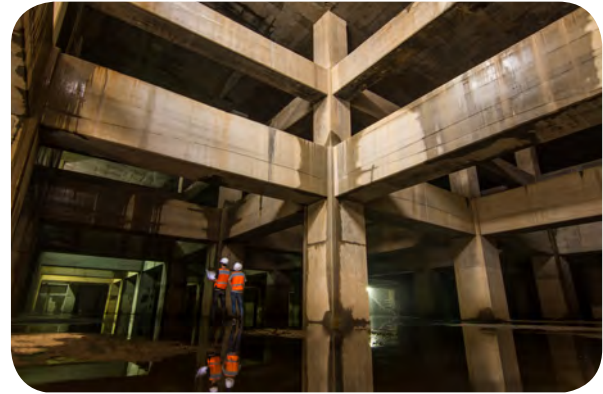
▲ Flood detention pond at the military police camp on Xinhai Road, Wenshan District
