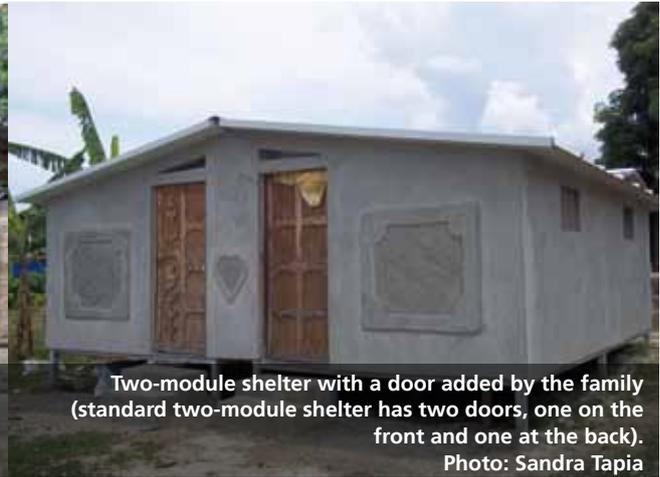
Two-module shelter with a door added by the family (standard two-module shelter has two doors, one on the front and one at the back).
