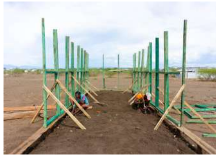
Right: Type E Pilot Shelter Construction - Frame Construction Process. © UN-Habitat
