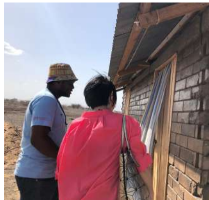
UNIC Director visits Shigeru Ban's durable shelter pilot construction. © UN-Habitat
