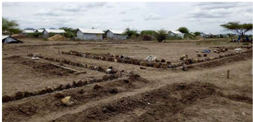
Bottom right: Temporary demarcation of plots using stones, in Village 2's Public Space construction. © UN-Habitat
