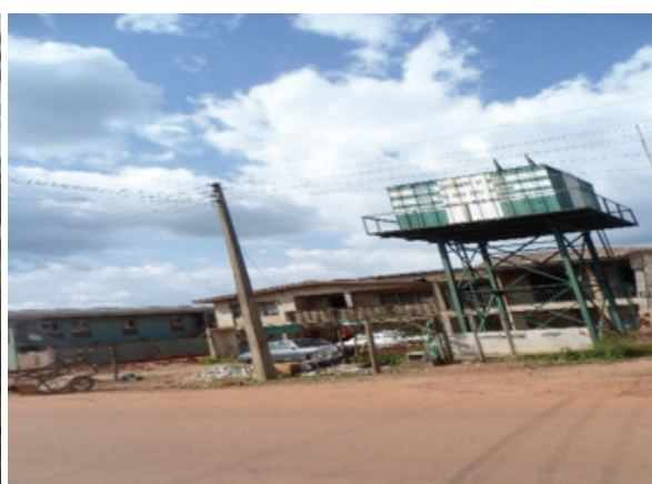
Plate 9: Public Water Supply in Ikirun Planning Area
