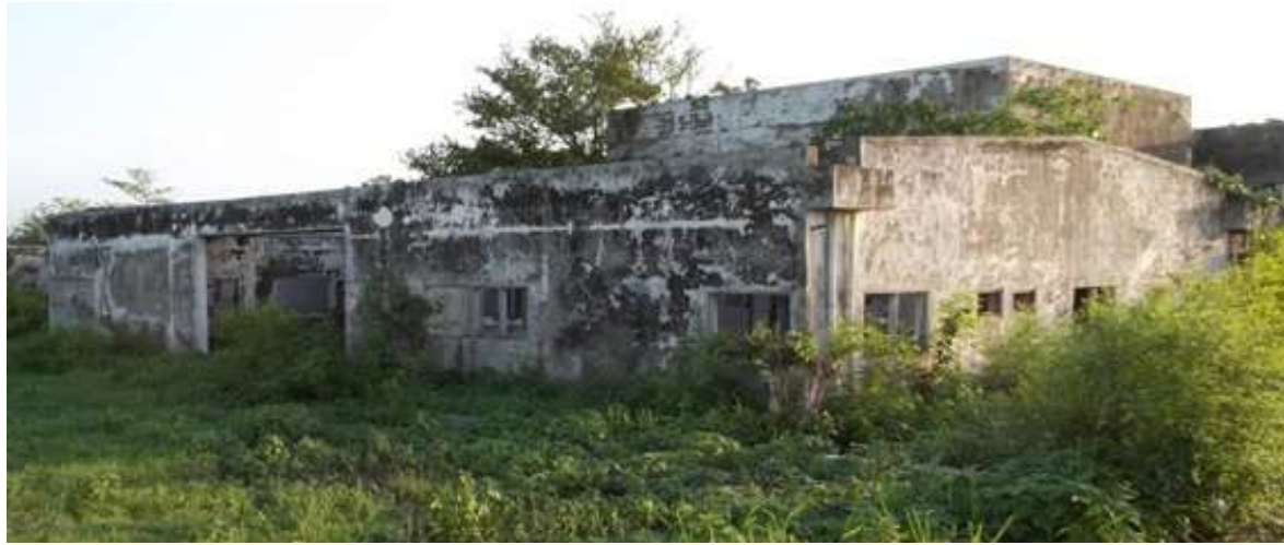
Plate 34: Derelict Ikire General Hospital complex on Ife-Ibadan Expressway
