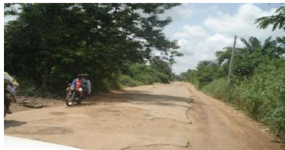
Plates 35 - 36: Poor condition of some roads in Ikire Planning Area
