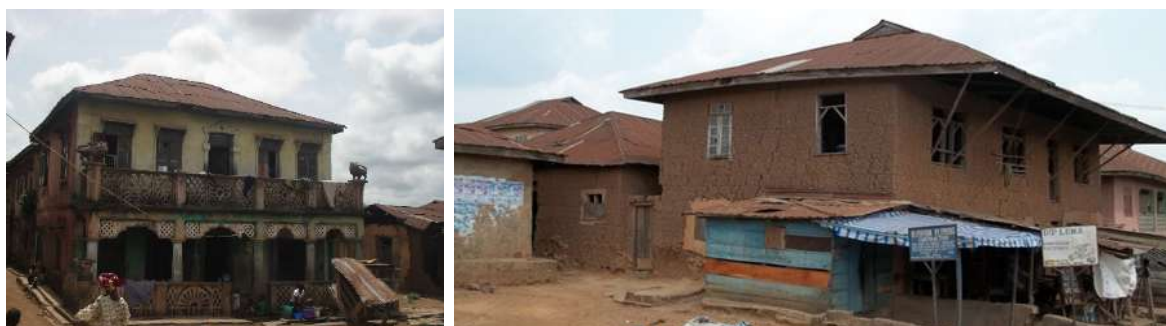
Plates 9 - 10: Residential Buildings in the core area of Ikire
