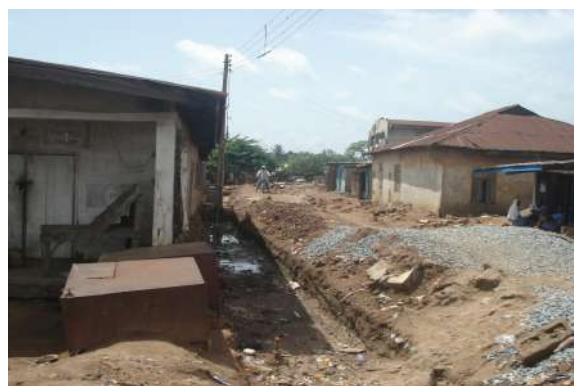
Plates 29 - 30: Blocked Drainage and new channel under construction in Ikire
