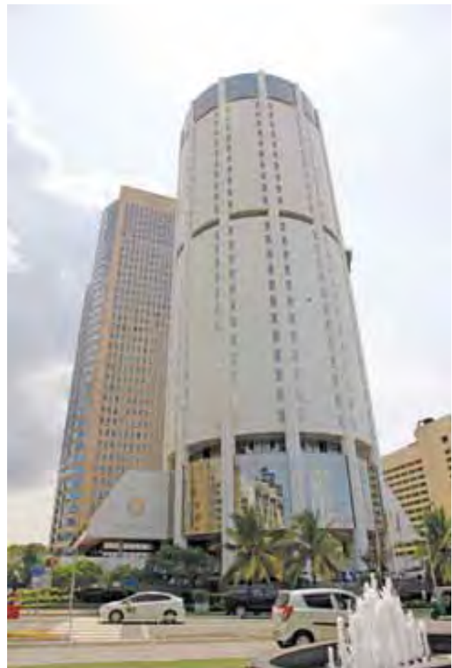
The iconic Bank of Ceylon building in Colombo's Central Business District
