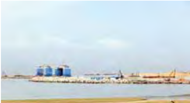
Fig 2.12: Port City current construction and future plan (L-R)
