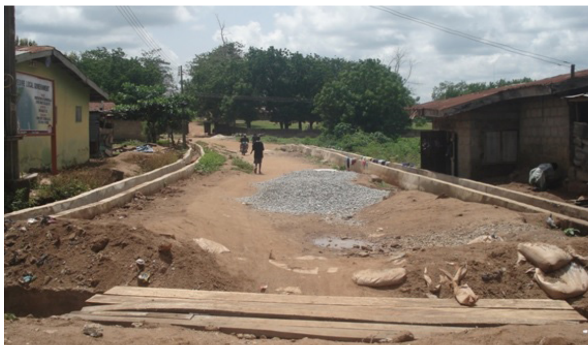
Plate 23: Road under reconstruction with provision of drainage channels in Iwo
