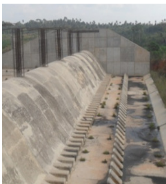
Plate 14: The spillway section of the Ile-Ife Water Supply Project under construction Source: Osun Structure Plan Survey, 2013
