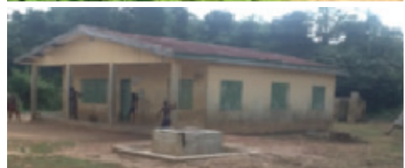
Plates 14 - 16: Water Supply Facilities in Ila-Orangun and Environs. Source: Consultants Survey, 2013
