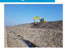
Yangon City, Myanmar: Emergency rehabilitation and stabilization of largest dump site (120 ha) after fire broke out in April 2018. Fire walls, water and leachate drainage construction in process.
