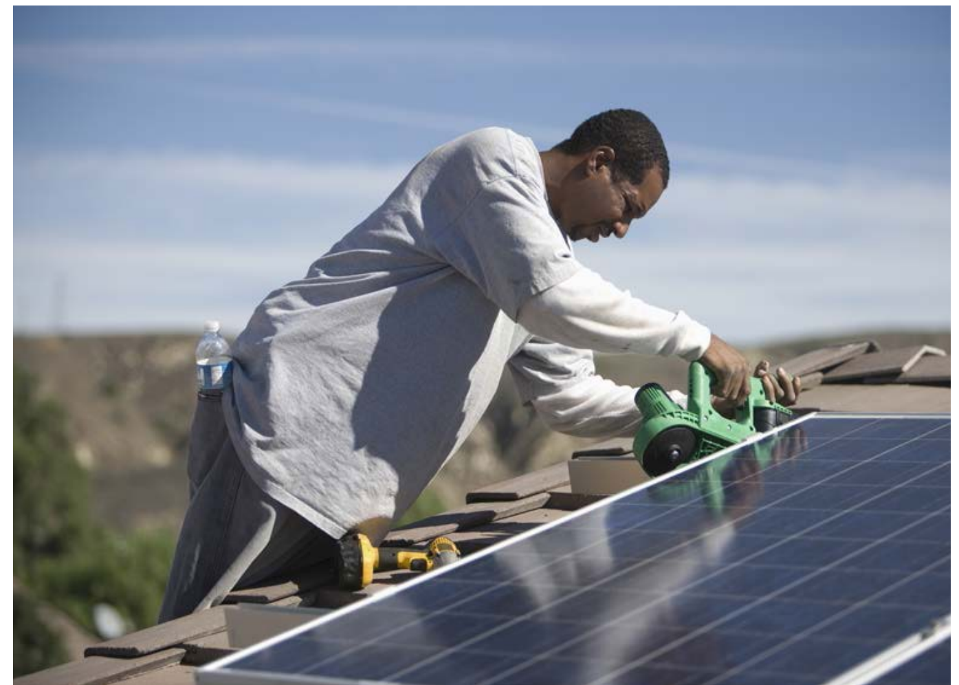
Fig.5: Installation of standalone photovoltaic panels as an alternative approach to increase access to electricity
