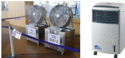
**Life time:** Compared to closed cycle air conditioning systems, these evaporative coolers have a much longer lifetime. However, the cleaning demand of evaporative coolers is higher.
