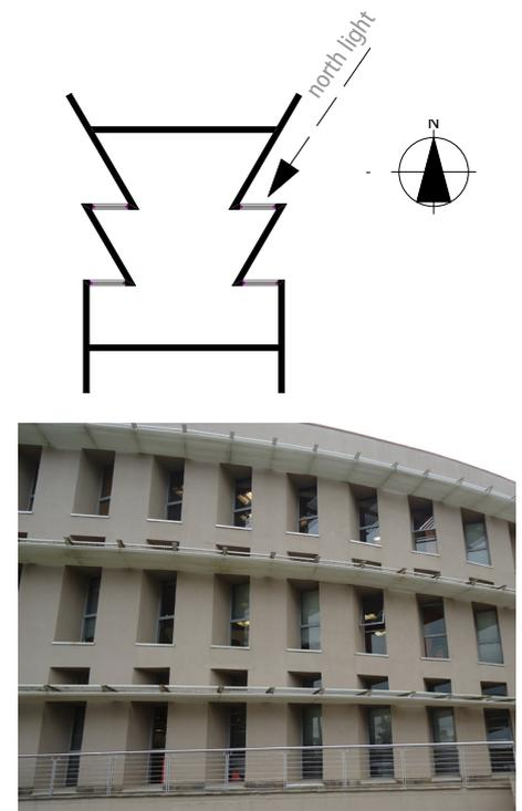
Windows are deeply recessed and oriented north to prevent direct solar radiation
