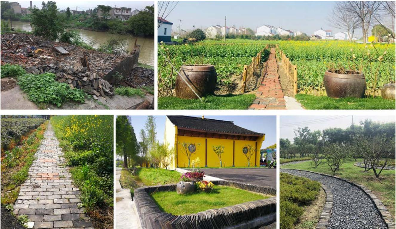
Fig. 3.42 Recycle building waste for pavement and landscape elements
