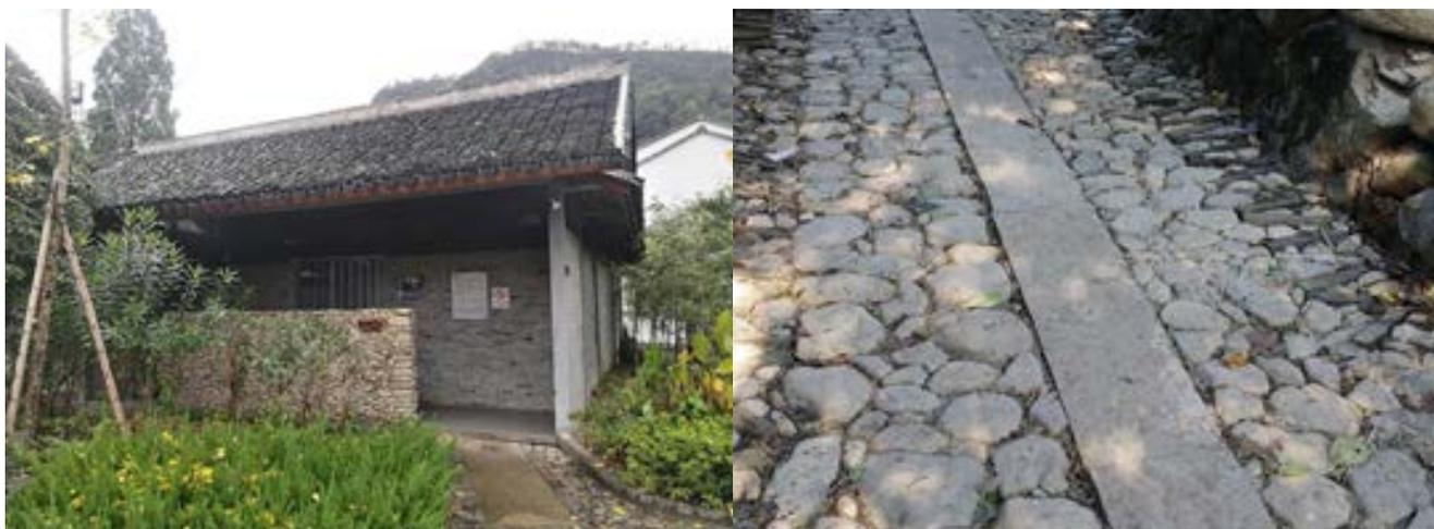
Fig. 3.15 The permeable surface of a walkway to an ecological public restrooms
