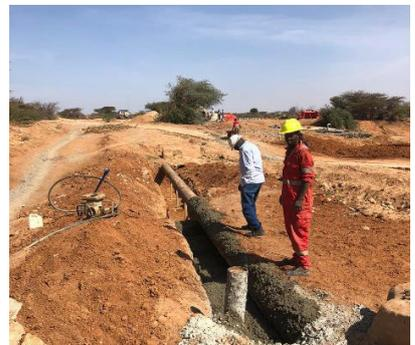
Erosion and flood protection works along critical point of the new pipeline: installation of flood retention walls, gabions, and protection of pipeline sections © UN-Habitat
