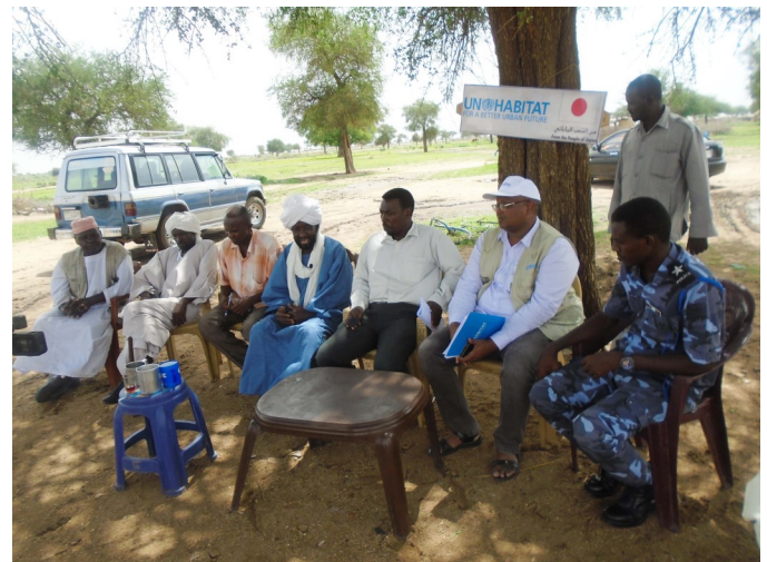
Handover of the construction site of public latrines to the contractor in the presence of community leaders and administrative representatives from the locality (2019)
