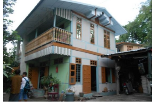
Figure (5) Brick Nogging Building Type
