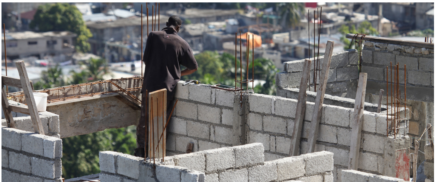
Ongoing construction Port-au-Prince, Haiti © UN-Habitat.
