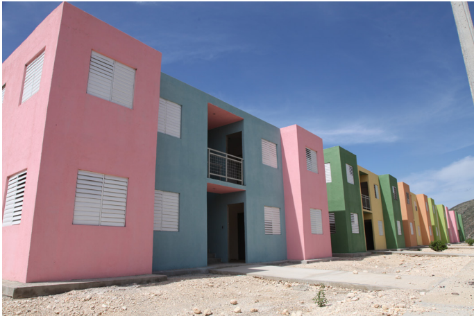
Government buildings project, Port-au-Prince, Haiti © UN-Habitat / Julius Mwelu.
