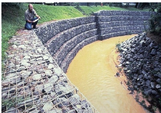
Controlling flood water using Gabions © gabions.co.nz.
