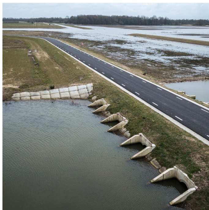
Dike reopens floodplain of the Rhine River © Joris van Gennip / The GroundTruth Project.
