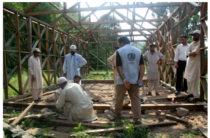
Reconstruction of a house in Bagh, Pakistan. © UN-Habitat.
