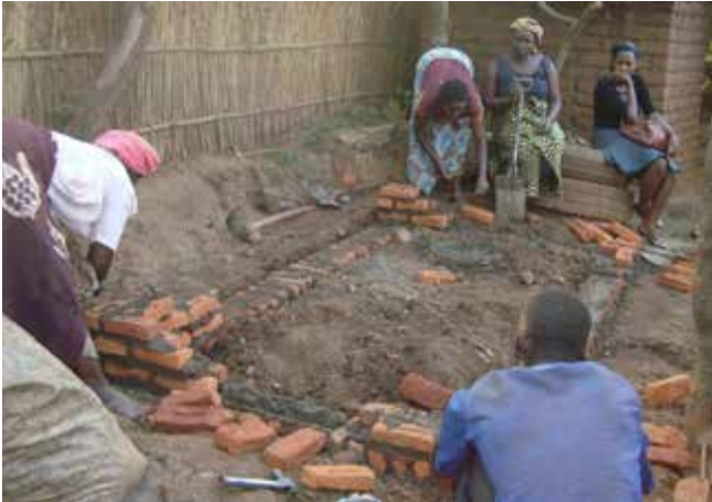
Ga Mashie Community house during upgrading. © UN-Habitat.
