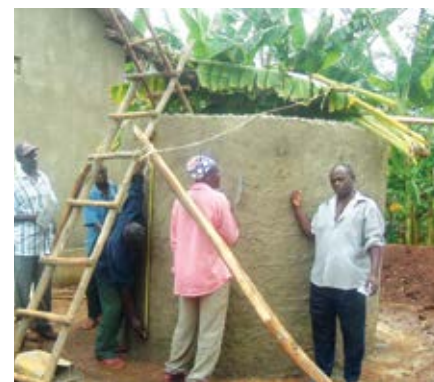
Construction of the rainwater harvesting tank. © UN-Habitat
