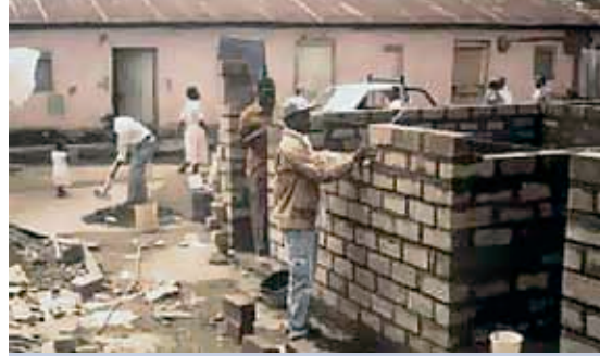
Figure 6: Artisans in Kenya constructing rental housing using stabilized soil blocks © UN-HABITAT
