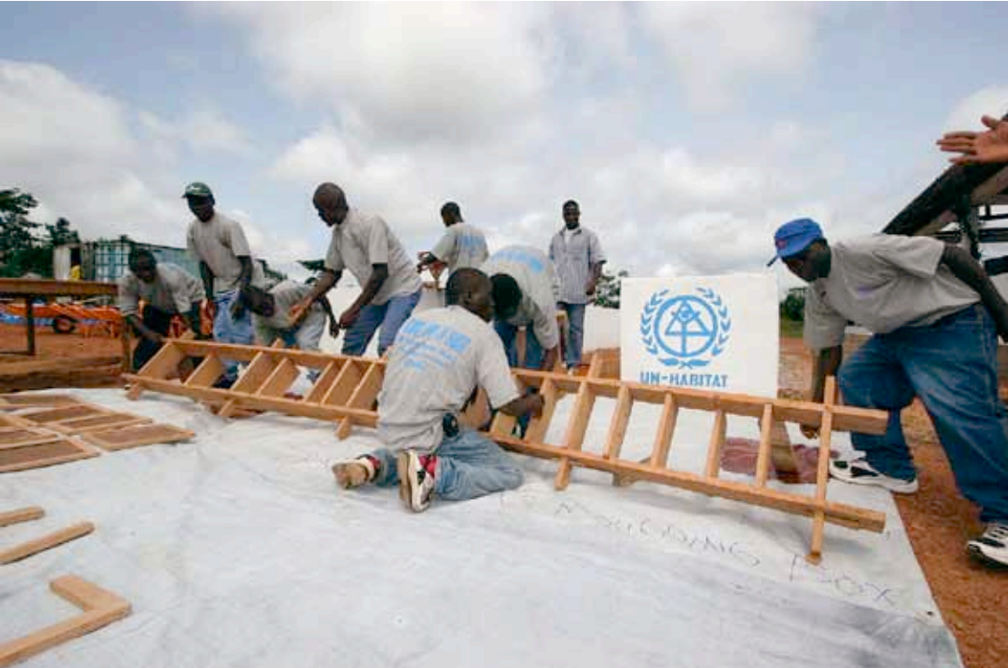
UN-HABITAT sponsored shelter construction in Liberia © UN-HABITAT
