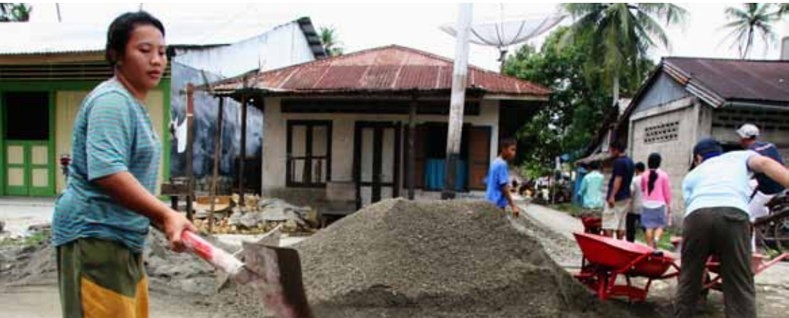
Collective self-help housing construction © UN-HABITAT
