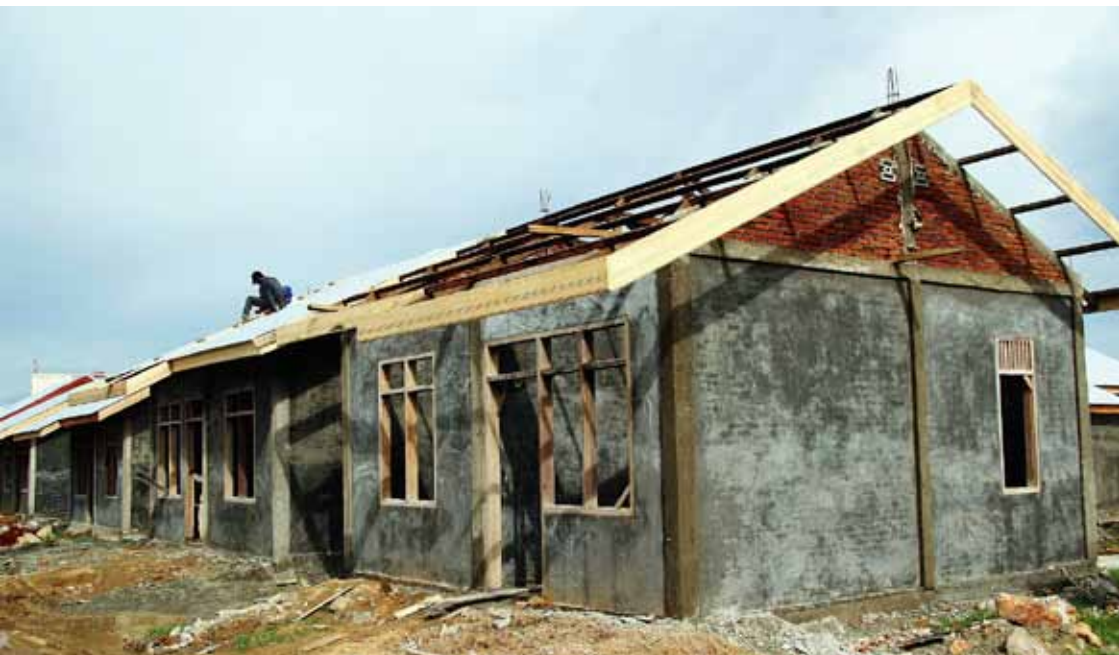
Housing reconstruction in Banda Aceh, Indonesia © UN-HABITAT
