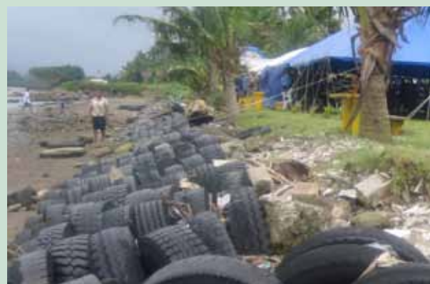
Coastal protection structures in Lami, Fiji © UN-Habitat
