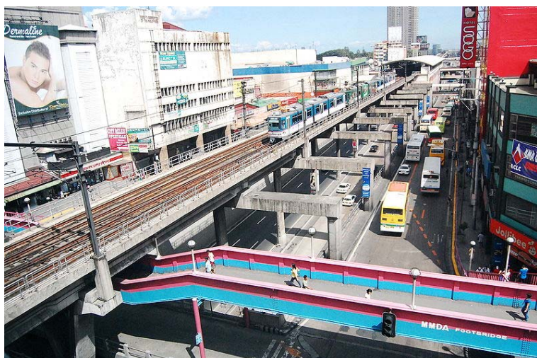
Figure 5. Metro Rail Transit (MRT-3) at Metro Manila (the Philippines)
