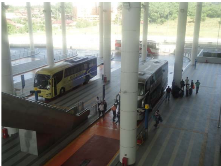
Figure 22. Integrated bus hub in Kuala Lumpur, Malaysia
