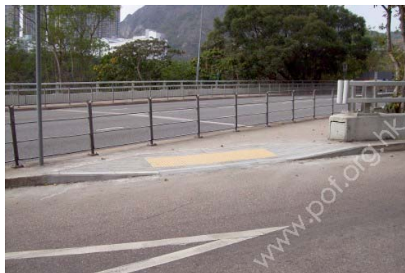
Figure 36. Slope in urban road curb in Hong Kong SAR
