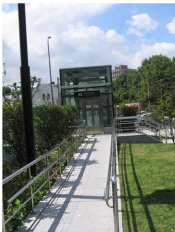
Figure 35. Barrier free facility at metro station entrance in Shanghai
