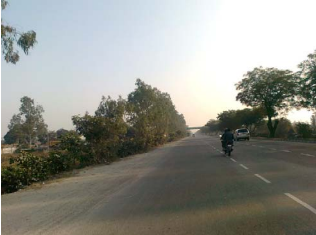
Figure 5. Location # 1, Site photograph
