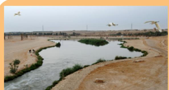
*Figure 10: The flood performance of the channel is improved by reprofiling and regrading Credit: Aga Khan Award for Architecture / Arriyadh Development Authority*
