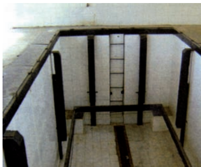
d) Pit for receiving container; note tiled surfaces, drain and weigh cells in corners
