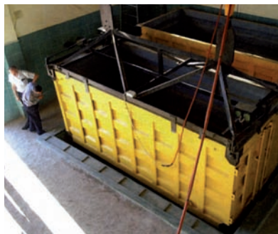
e) Container being lowered into pit
