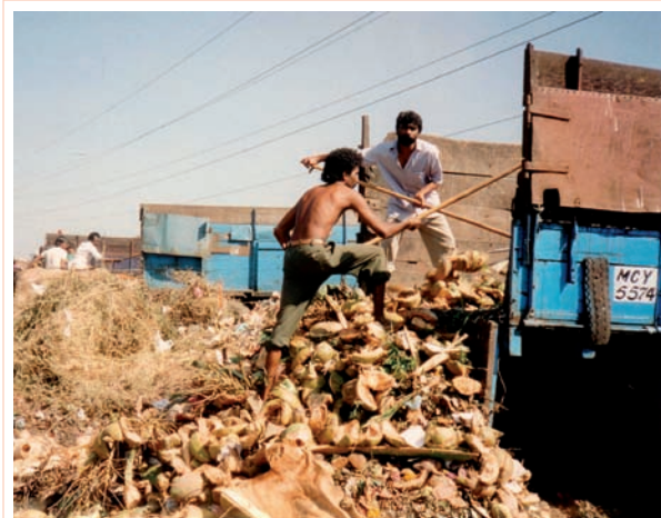
Photo 7.11 Manual unloading of rigid truck at disposal site
