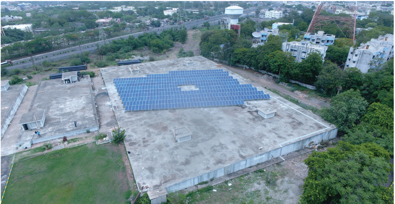
Rajkot, India, and Urban-LEDS project city, has installed a 145kWp solar PV system to help power its Aji water treatment plant
