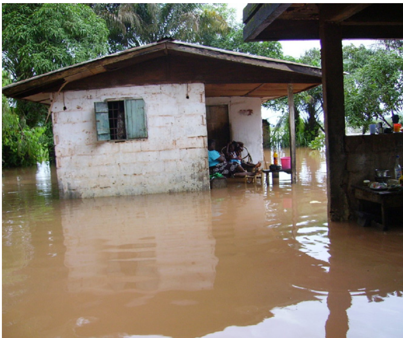
Floods in Congotown, Liberia © UN-Habitat
