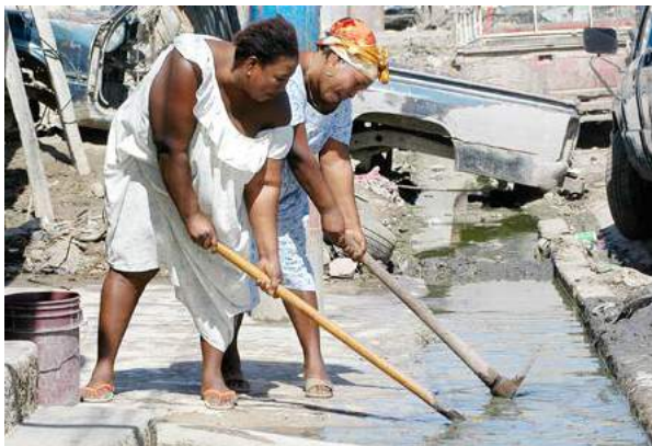
Women clearing drains after flooding in Peru. Source: IFRC.
