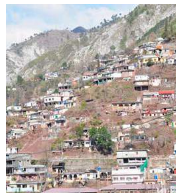
Urbanization on land identified as extremely hazardous. Source: UCL.
