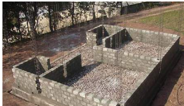
Model house constructed to generate training and information materials. Rising wall and steel reinforcement in confined masonry construction. Source: UN-Habitat.
