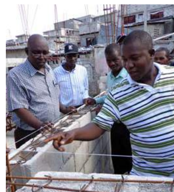
Government engineer on site at weekend event demonstrating standards for steel reinforcement.
