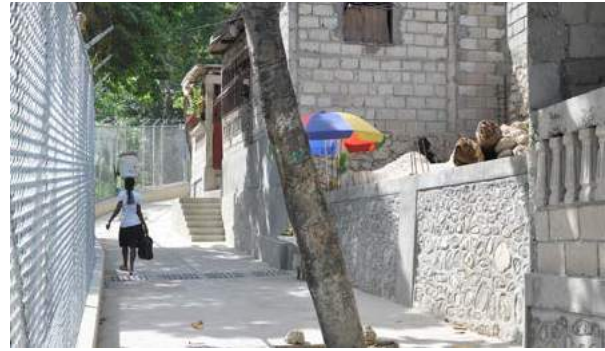
Ravine in informal neighbourhood of Campeche after investment in improvement measures to improve circulation and drainage, and to reduce solid waste disposal and flooding risk. Upgrading infrastructure in residential neighbourhoods supported housing and settlement recovery. Source: UCL.
