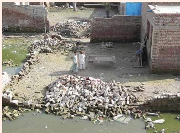
Flood recovery involved rehabilitation of boundary walls and improved area planning and drainage. Source: UN-Habitat.
