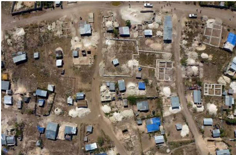
Reconstruction after the earthquake in Haiti, materials on site and most houses under construction at the same time. Source: APDER.
