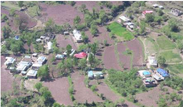
Rural houses reconstructed 4 years after Kashmir earthquake. Over 90 percent compliant with safer building standards. Source: UN-Habitat.
