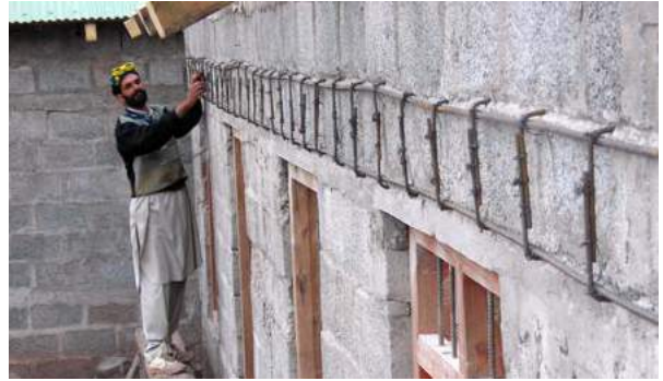
Retrofitting an external band to make substandard new construction safer. Technical assistance to diagnose and address emerging problems. Source: UN-Habitat.
