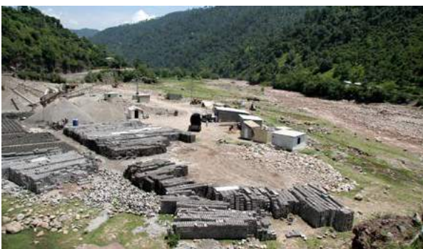
Expansion of concrete block production capacity to meet increased demand in reconstruction. Source: UN-Habitat.
