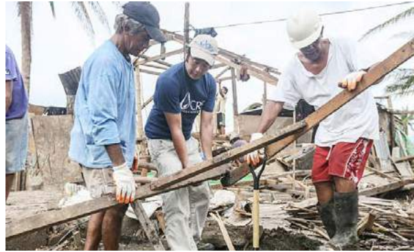
Dismantling damaged houses and salvaging materials after cyclone Haiyan (Yolanda). Source: CRS.
