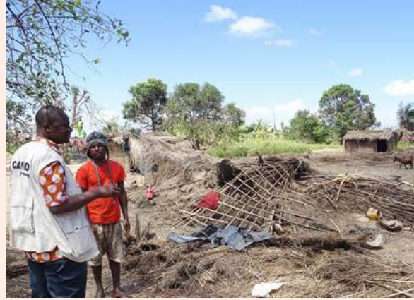
Major damage from cyclone Idai in Mozambique caused extensive agricultural losses to livelihoods and required complete reconstruction. Source: CRS.
