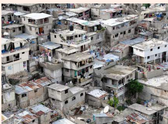
Existing informal neighbourhood, increasing in population and density after the earthquake with added floors and other extensions. All pre-earthquake buildings. This is also the site of recovery as many earthquake-affected families moved to this neighbourhood to rent a new home. Technical assistance is also required in neighbourhoods that are not destroyed. Haiti. Jalousie. Source: UN-Habitat.
