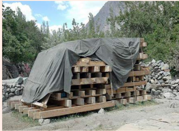
Roof timbers removed from flooded houses and stored for reuse in Hunza. Good quality timber is scarce in the area and very valuable. Source: UN-Habitat.
