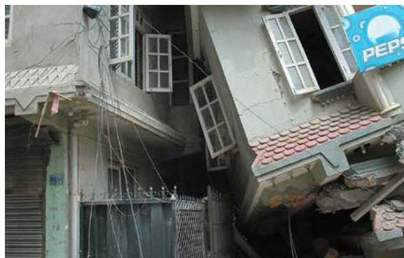
Individual building collapse in Kathmandu after the 2015 earthquake and damaged caused to the neighbouring building. Property insurance in urban areas needs to take account of settlement as well as building and risk factors. Source: Shelter Cluster Nepal.
