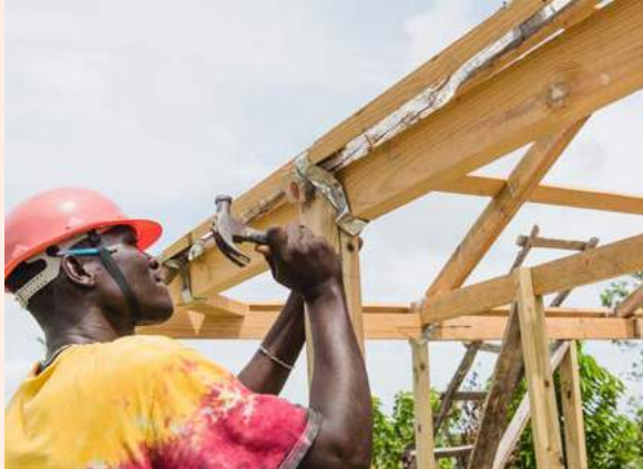
Carpenter installs hurricane straps. Source: CRS.
