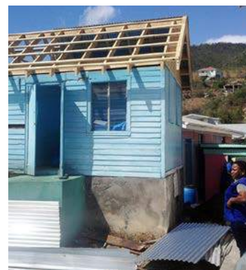
Rebuilding local timber framed house after Hurricane Maria, Dominica.
