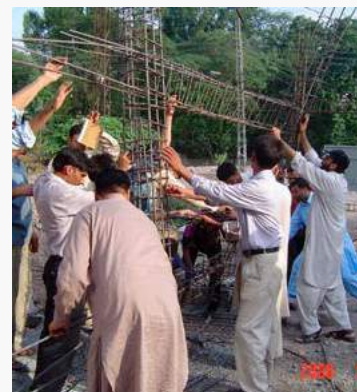
Practical steel fixing training on a temporary open site. Source: GOAL.
