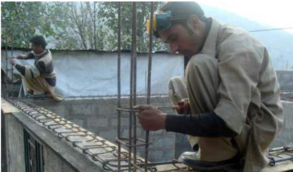
Technical assistance mobile steel fixer demonstrates steel band corner details at lintel level for household and masons to replicate. Source: UN-Habitat.
