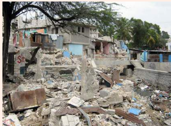
Damage in the neighbourhood of Ravine Pintade after the 2010 earthquake in Port-au-Prince. Source: Global Communities.
