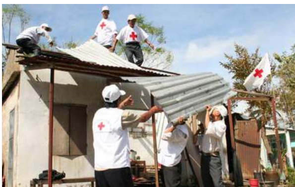
Red Cross team helps with repairs to roof to make the house habitable after cyclone damage, Vanuatu. Source: IFRC.
