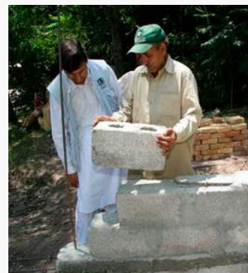
On-site advice to masons.
