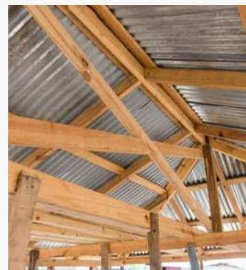
Strengthening roofs in Caribbean to avoid recurring damage in hurricanes. Source: CRS.
