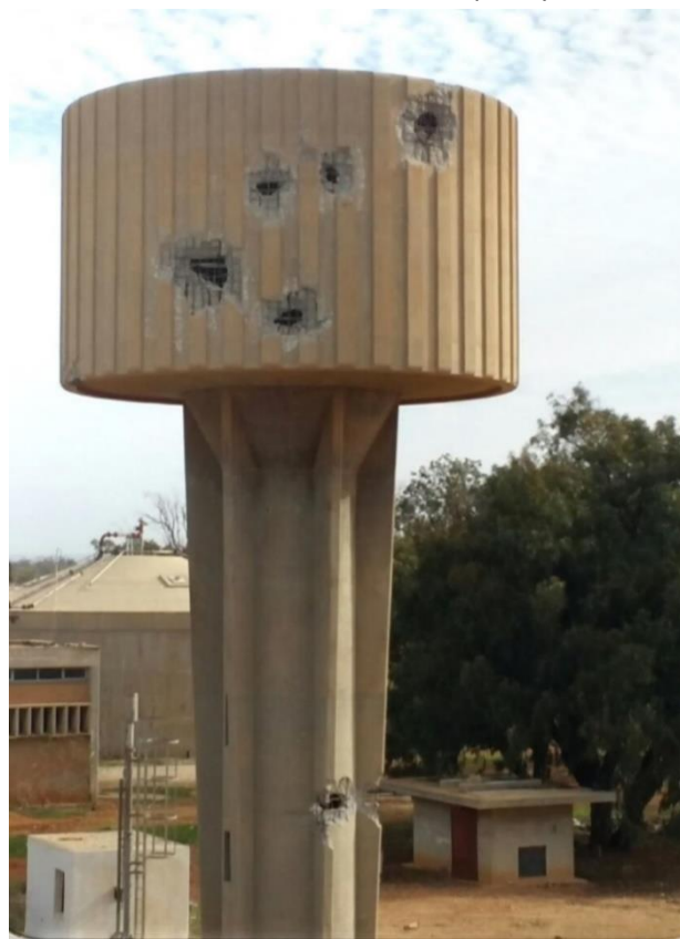
Damage in Benina services building, Courtesy: General Co for Water and Sanitation
