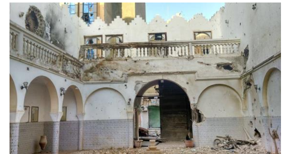
Former and present situation of the cultural house Source: Key informants
