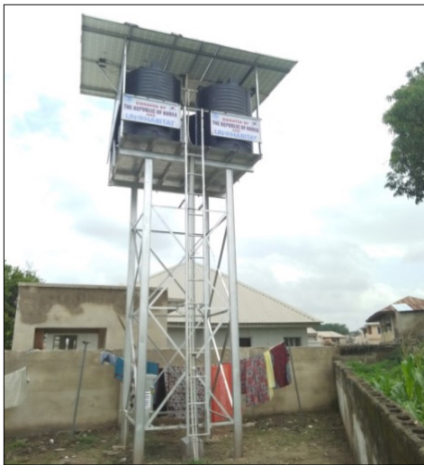
» Smart-Metered Solar Borehole in Niger State (Nigeria)
