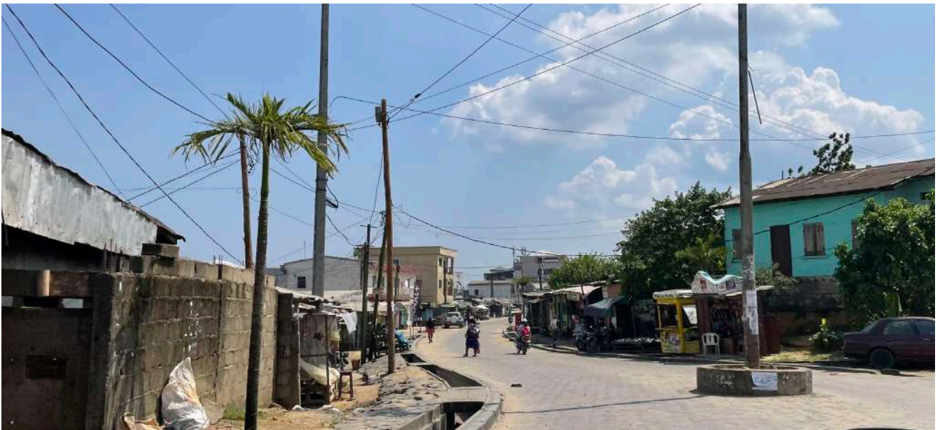
Photo 19. One of the secondary roads in Mambanda, paved with semi-permeable paving materials Source: UN-Habitat
