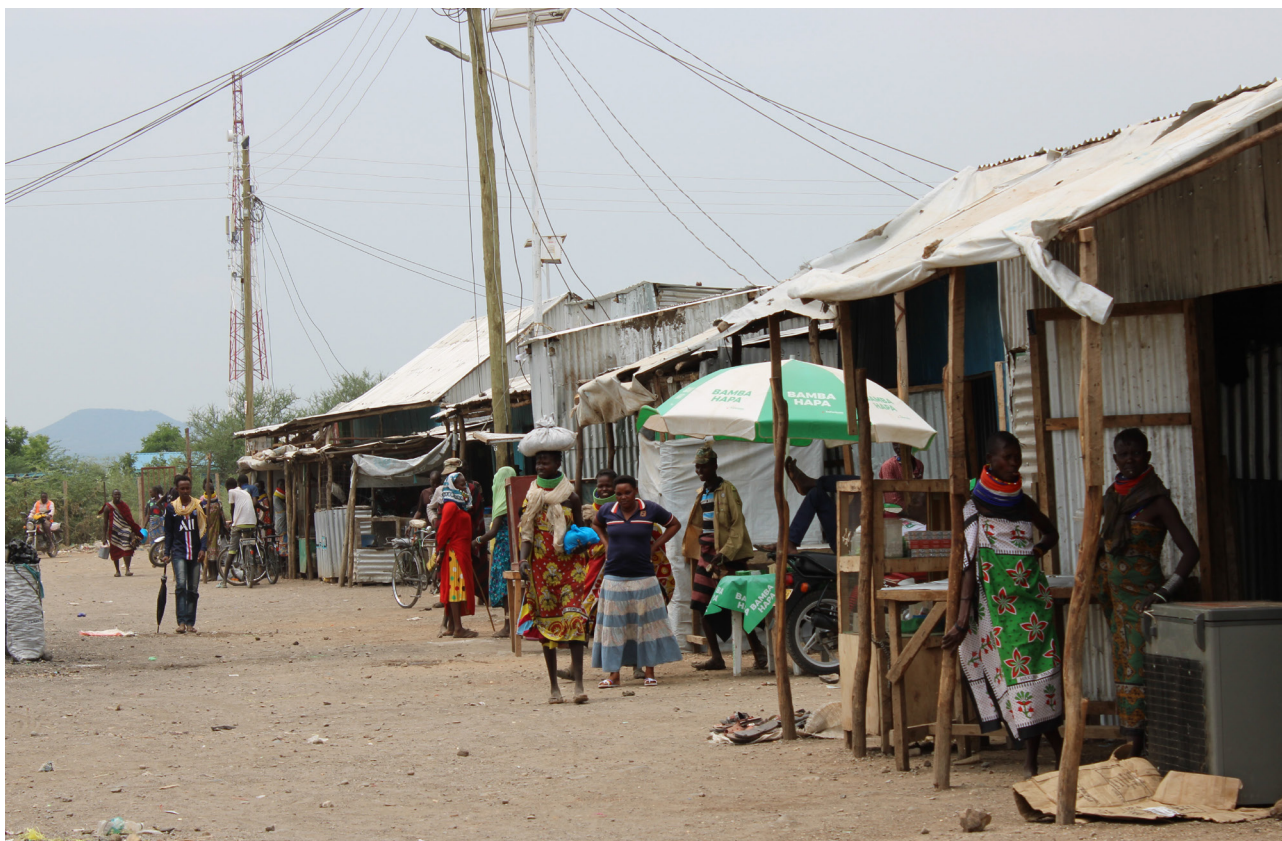
Communication Infrastructure in Kakuma-Kalobeyei. © Baraka Mwau
