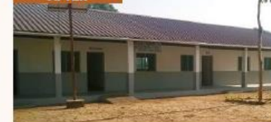
UN-Habitat cyclone resilient design used to rebuild schools in Namputua District, Mozambique ©UN-Habitat
