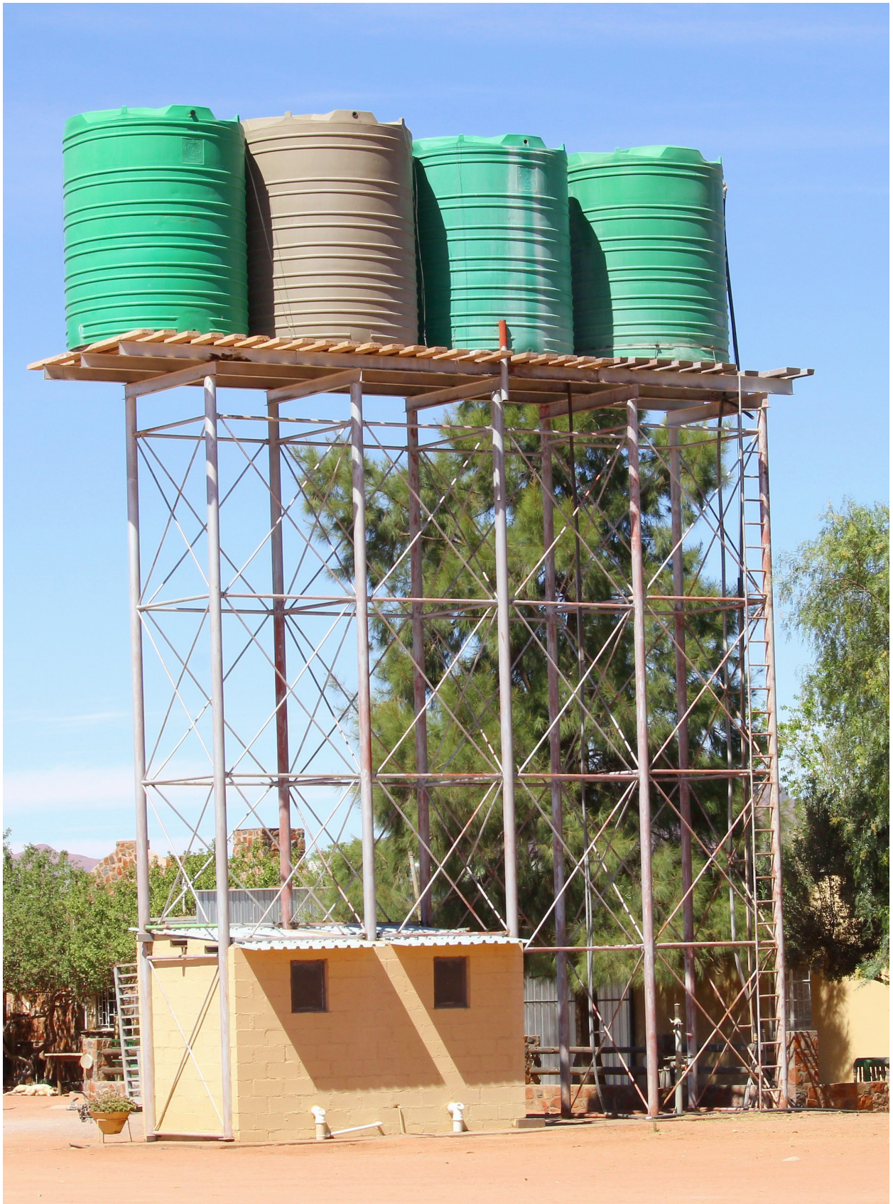
Rainwater harvesting in storage tanks, public drinking water distribution in Namibia, southern Africa. © Shutterstock/ingehogenbiji
