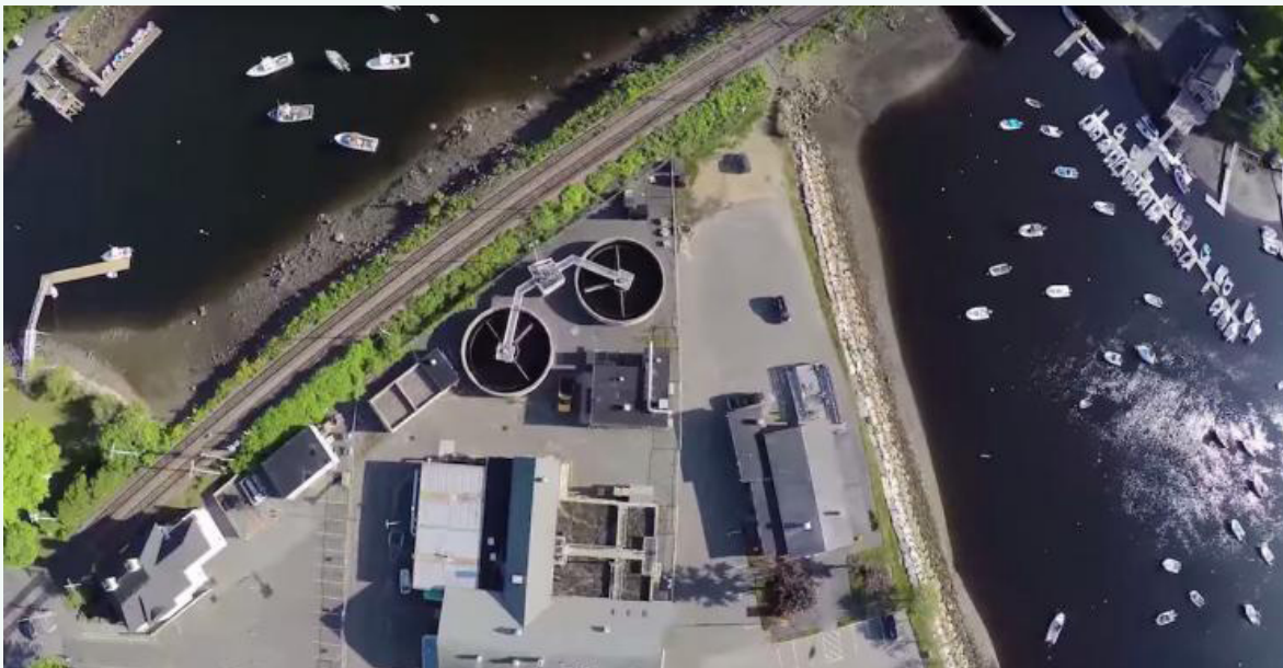
This aerial view of the wastewater treatment plant emphasizes how the site is exposed to water on two sides.
