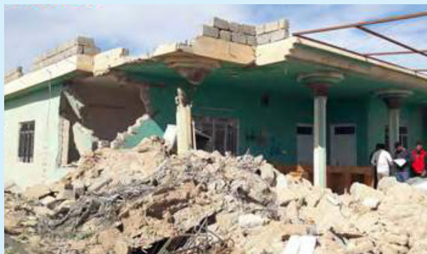
Figure 7: Housing rehabilitation in Sinjar, Iraq (before). Photo: © UN-Habitat
