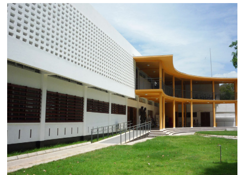
Perforated walls and louvers for shading and ventilation © Tengbom Architects
