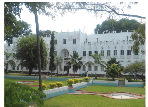
Light coloured external finishes
