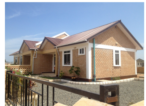
Orientation along east-west axis. Local building materials © UN-Habitat / Marja Edelman
