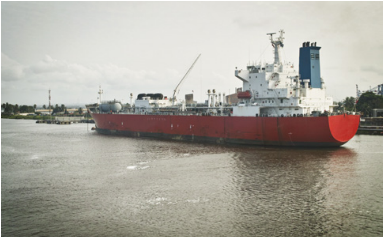
Abidjan's port infrastructure contributes to good connectivity with other Western African states but it would benefit from digitalization to ease congestion
