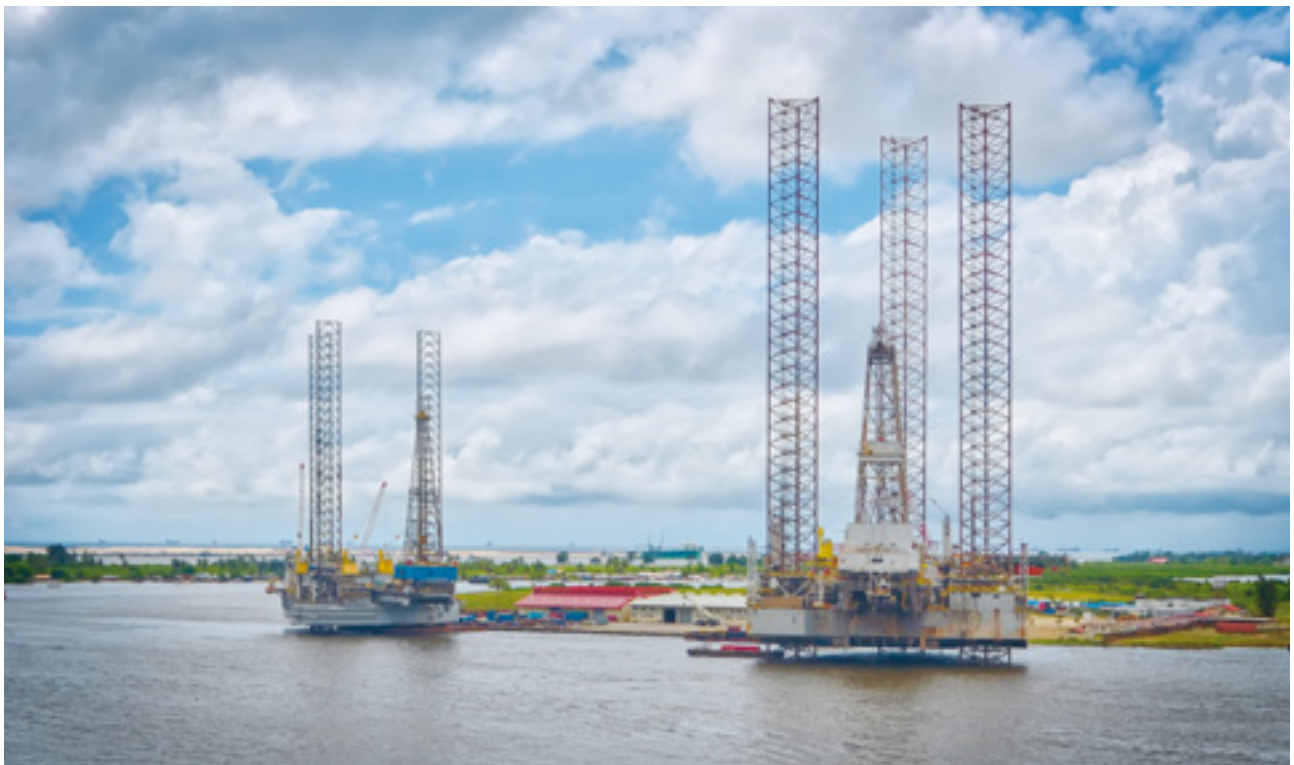
An oil refinery in the Port of Lagos. Africa's major oil rich countries such as Nigeria take the lead in resources FDI
