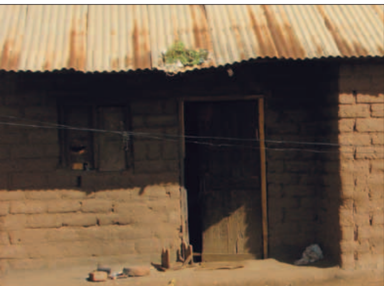
Figure 44. Very low-cost adobe brick construction in a THA in Lilongwe
