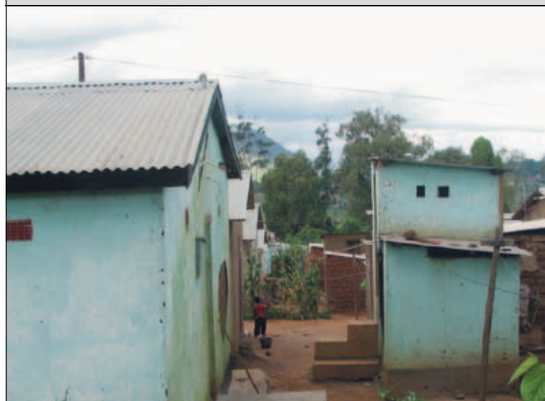
Figure 17. Ecosan latrine and bathroom blocks in CCODE, Blantyre
