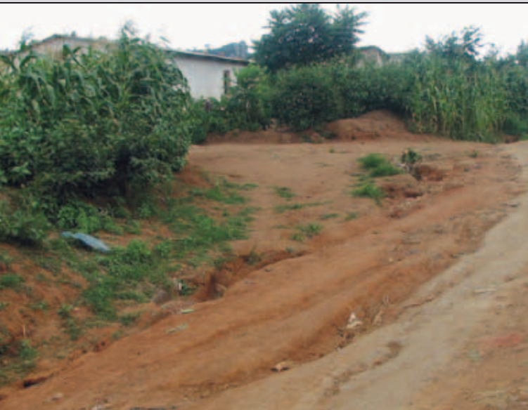
Figure 42. Land cleared for a road, but not engineered Photo © Graham Tipple
