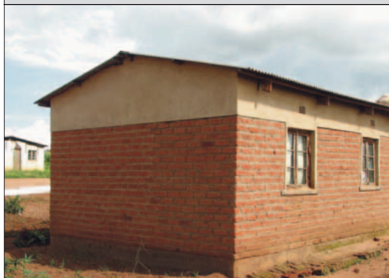
Figure 11. Habitat for Humanity dwelling in Area 49, Lilongwe Photo © Graham Tipple
