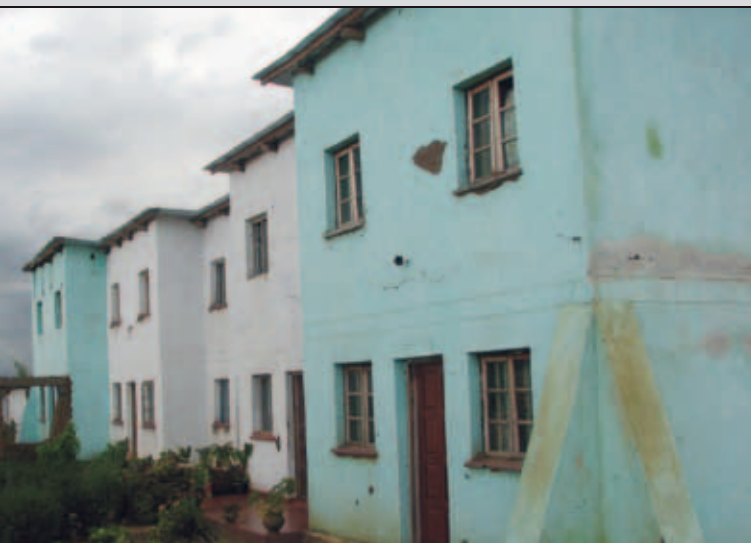
Figure 15. Two-storey experimental CCODE housing in Angelo Goveya, Blantyre
