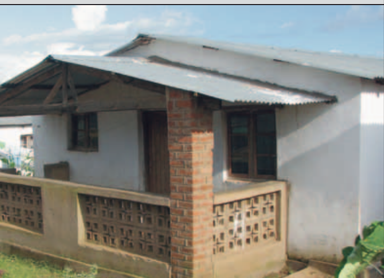
Figure 45. A porch which is a typical small improvement built by single artisans
