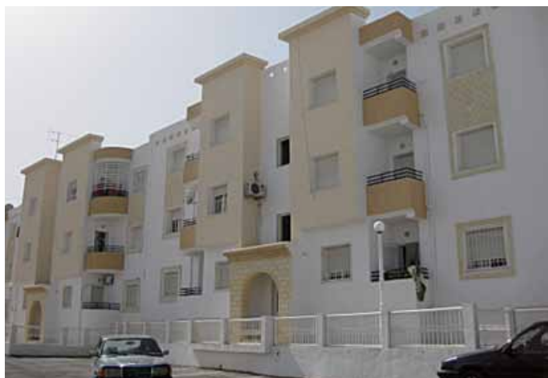
Figure 3.11 SNIT Low-rise apartments complex, Sidi Hussain, Tunis Photo © Tarek El-Sheikh
