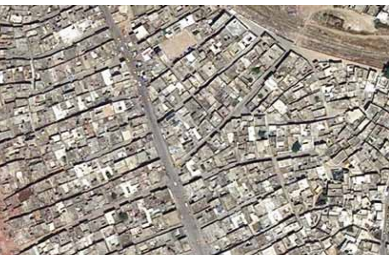
Figure 5.10 Sayeda Al Manoubia older informal area of single story houses in process of densification Source: Google Earth ©2011 Google Image, ©2011 Europa Technologies ©2011 Digital Globe, accessed 30 March 2011.
