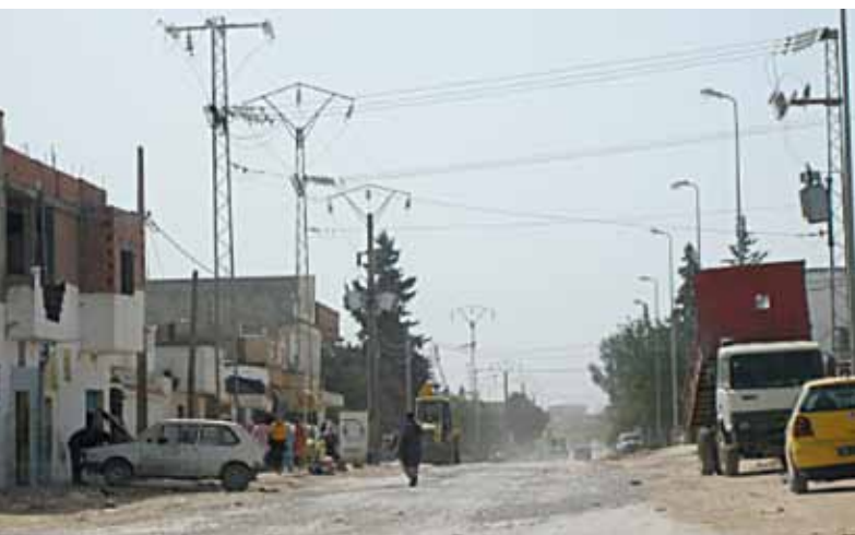
Figure 8.6 Overhead medium and low tension power distribution in informal area
