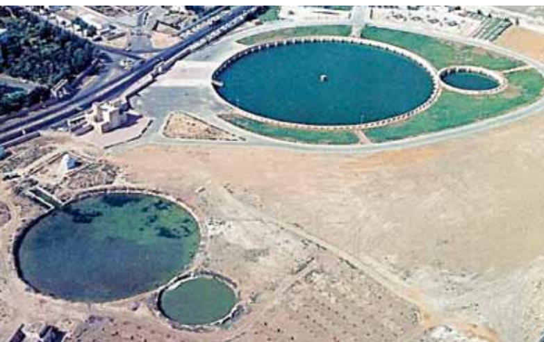
Figure 8.1 Old and new water purification plants
