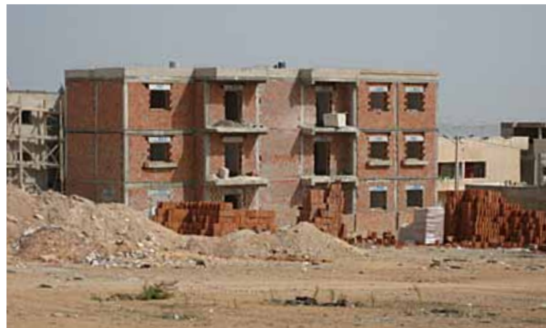
Figure 9.5 Example of RC concrete frame and extruded brick infill in social housing construction
