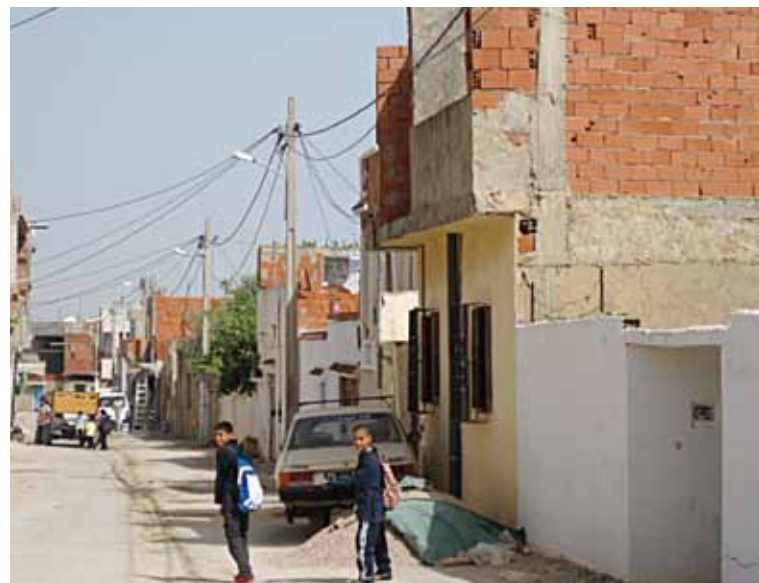
Figure 3.4 Densifying informal neighbourhood, Al Zohor Area Photo © Tarek El-Sheikh
