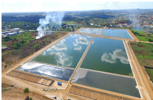
Figure 4.15: Ngwerere treatment ponds
