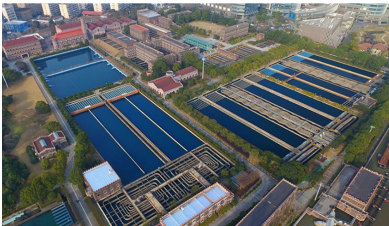
Figure 6.10: Aerial view of Yangshupu Waterworks
