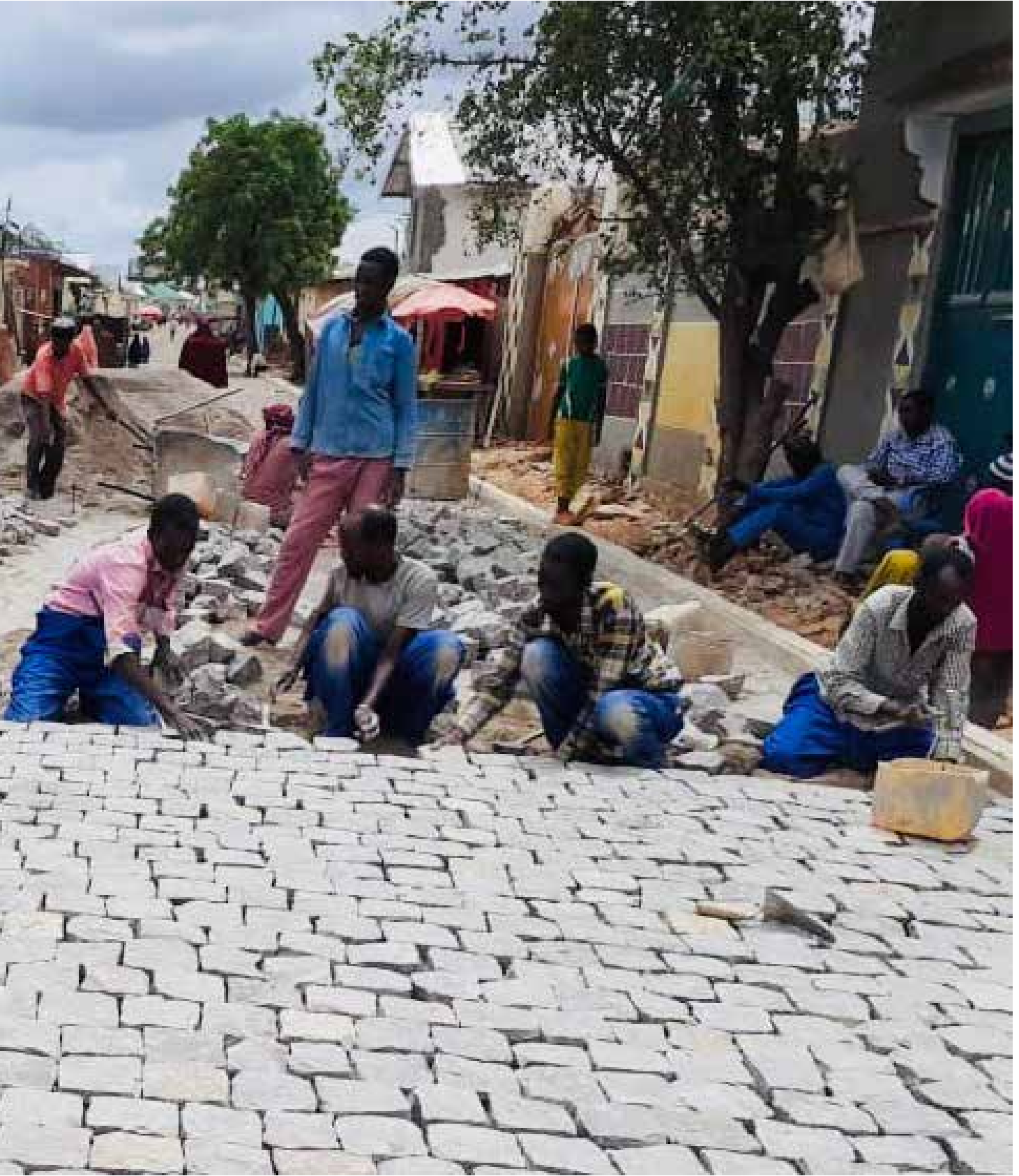
Fig. 53. Paving of internal road © Hiran Online
