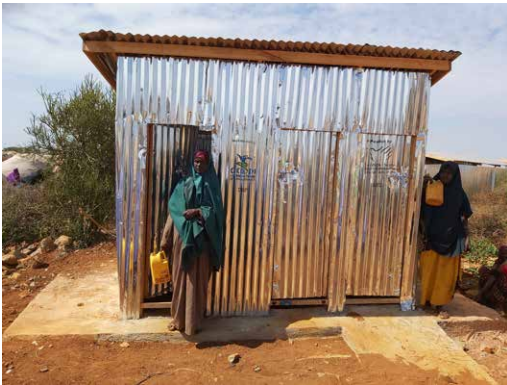
Fig. 33. New latrines for IDPs ©AICS
