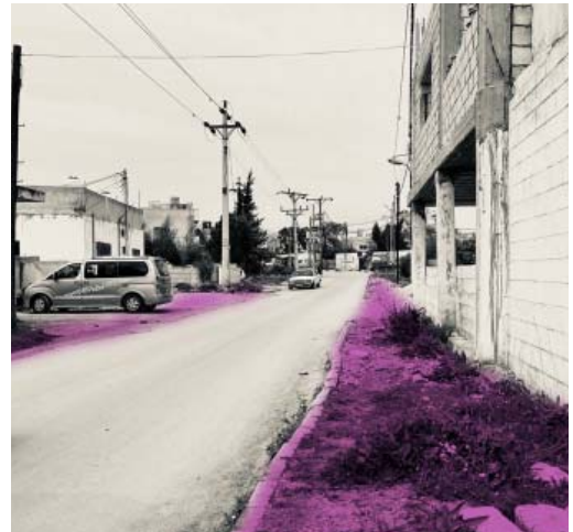
Lack of Sidewalks & Ruined Sidewalks
