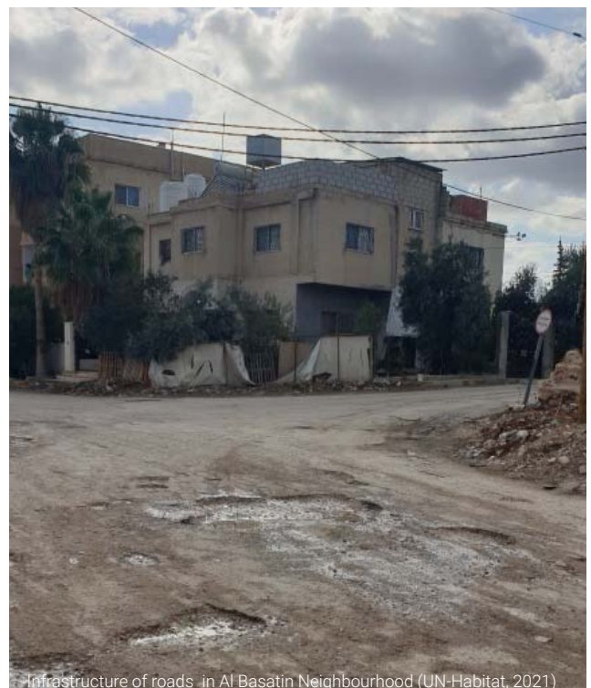
Infrastructure of roads in Al Basatin Neighbourhood (UN-Habitat, 2021)
