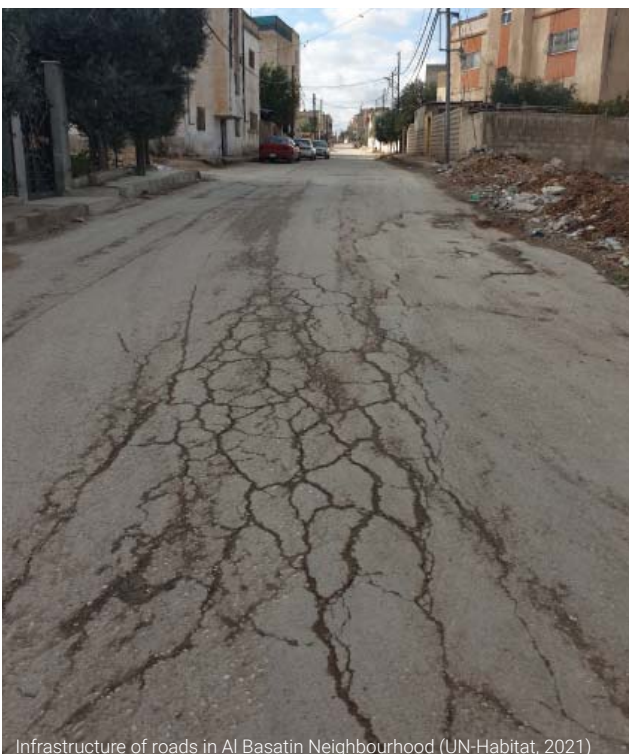
Infrastructure of roads in Al Basatin Neighbourhood (UN-Habitat, 2021)
