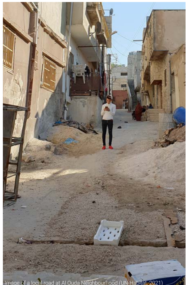
Image of a local road at Al Ouda Neighbourhood (UN-Habitat, 2021)
