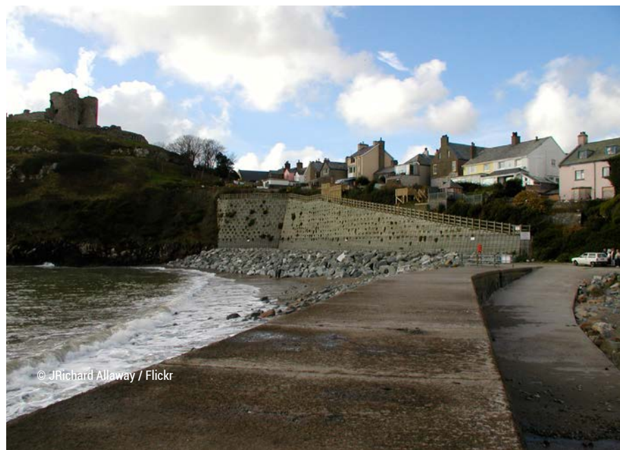
Figure 12: Coastal erosion management, Criccieth, North Wales, UK
