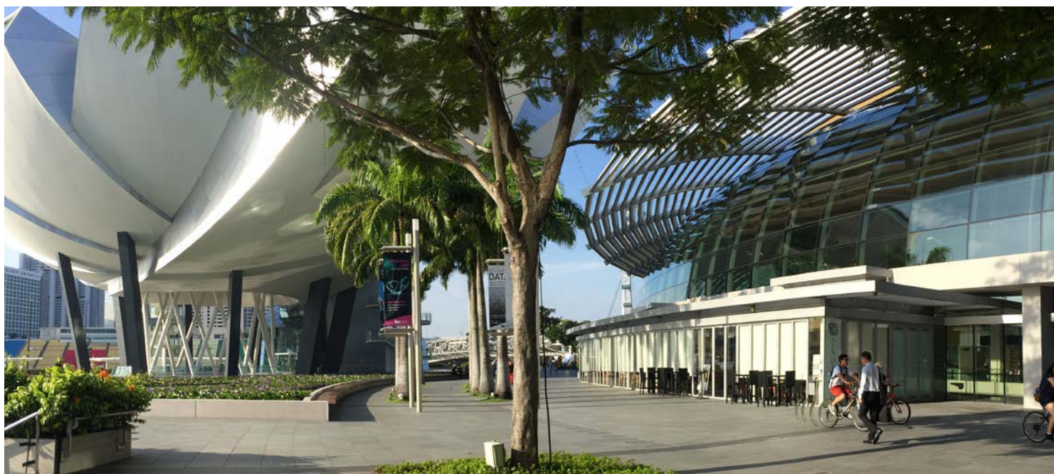
Figure 22: In Singapore, different uses and typologies intertwine in a well-established master plan.
