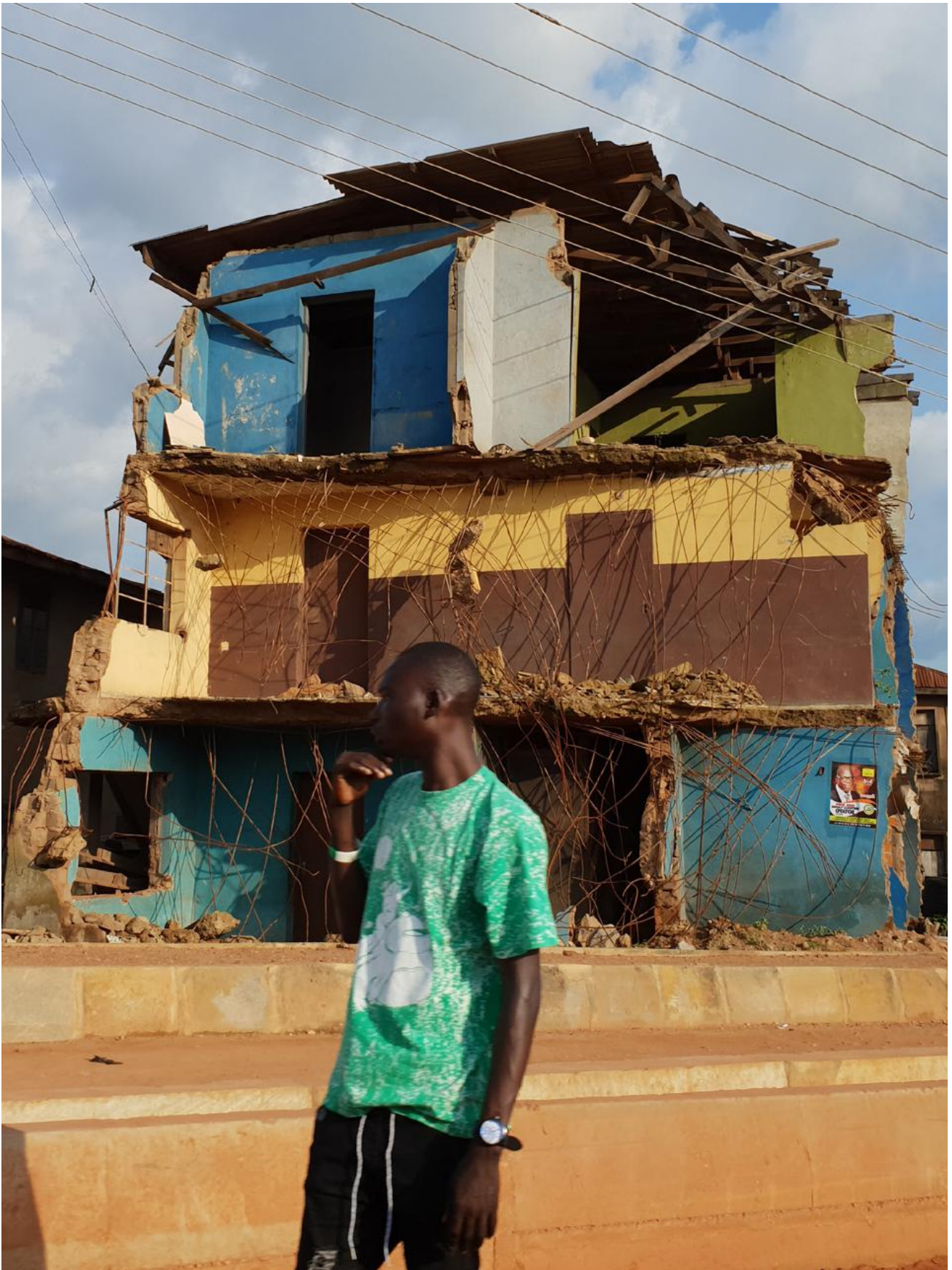
Fig. 15. Abeokuta House Demolitions © UN-HABITAT (2018) Francesco Tonnarelli
